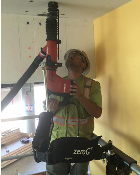
Vertical Drilling w/ Dust Extraction Ring tool Holder Stanford University Hospital
