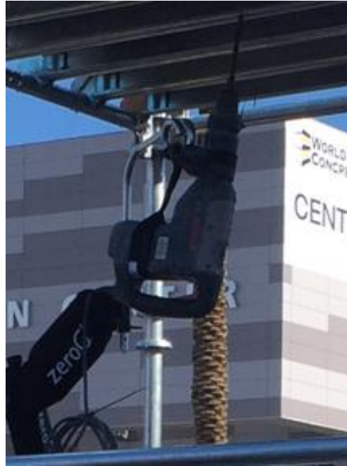
Vertical Drilling Sling Tool Holder
